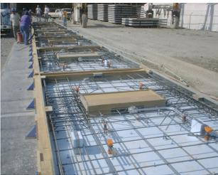
Precast concrete sandwich wall panels
