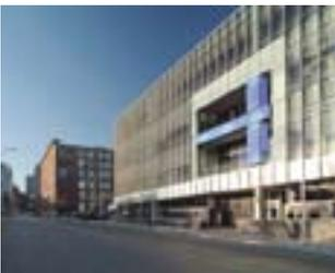
The precast concrete frame and many of the connections are intentionally visible through the glass.
