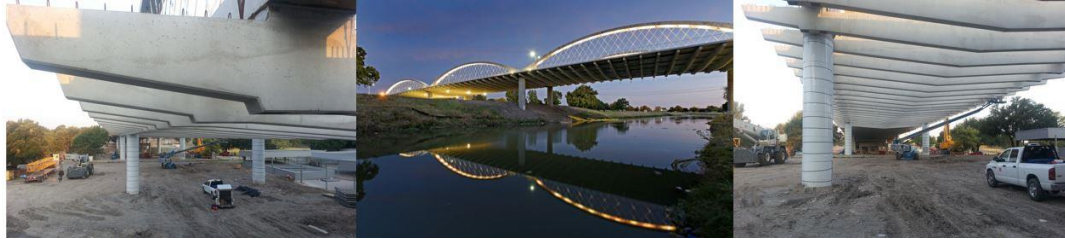
West 7 th Street Bridge – Fort Worth, TX photos by Adam Mainka, HEI Prod/Plant Manager
