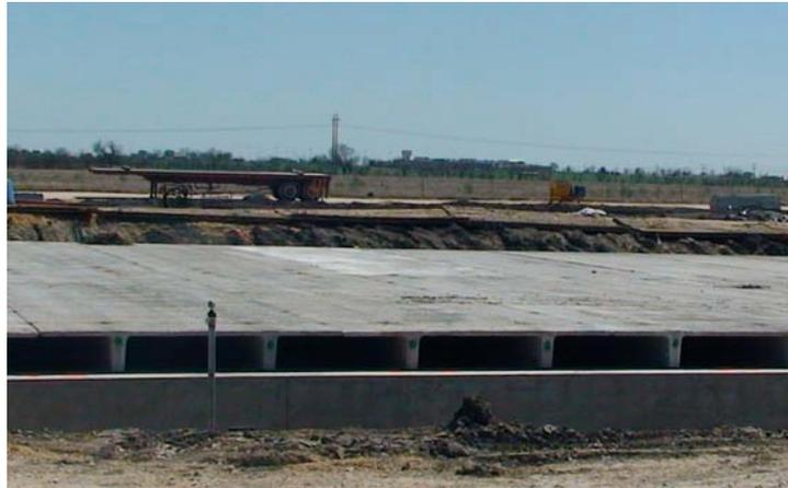
The heated storage building is approximately 28,500 sf and contains a large arms storage vault. The vault section was cast in place on precast grade beams. The rest of the structure was total precast construction utilizing precast grade beams with 24" double tee floor and roof.
