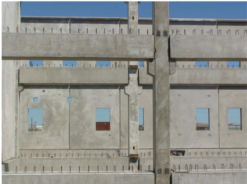
Heldenfels Enterprises began the fabrication of the components in January 2010. By the end of March 2010, all the precast pieces had been cast, erection of the main office building was complete and the OMS building was more than 50% complete. Precast Erectors, Inc. began erection in mid-February amid a pattern of rainfall that inundated the project site on an average of every 8 days.
