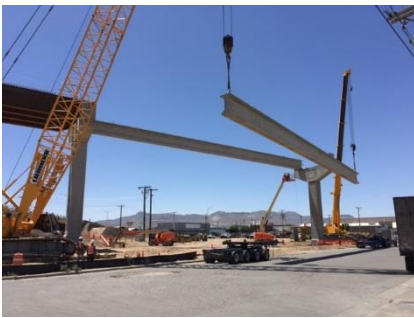
HEI produced TXDot TX-70 Beam installation @ Loop 375 Border Hwy West Extension, El Paso, TX Pictures by Adam Mainka, VP of Operations & GM, HEI El Paso Plant
