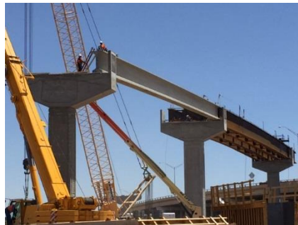
HEI produced TXDot TX-70 Beam installation @ Loop 375 Border Hwy West Extension, El Paso, TX Pictures by Adam Mainka, VP of Operations & GM, HEI El Paso Plant
