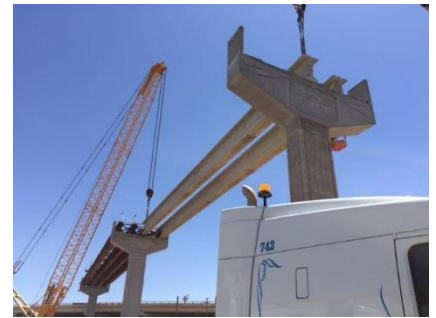
HEI produced TXDot TX-70 Beam installation @ Loop 375 Border Hwy West Extension, El Paso, TX Pictures by Adam Mainka, VP of Operations & GM, HEI El Paso Plant
