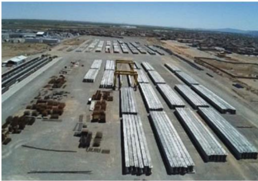
Heldenfels Enterprises Inc. opened a new prestressed concrete plant in El Paso, Tex., to help supply beams for the Loop 375 Border Highway West extension project, which includes 21 bridges. Courtesy of Heldenfels. PCI Journal | May-June 2017
