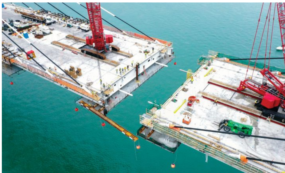
Main span bridge deck construction commenced December 2022 from opposite Detroit River banks. The Canada and U.S. crews methodically inched closer to each other, leading to May 2024 placement of the final precast deck slabs, followed by six weeks of mid-span closure beam erection and deck pours.
