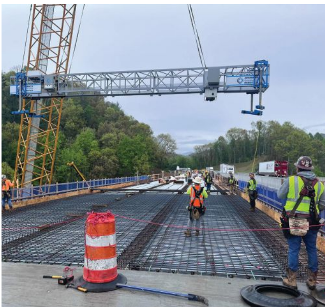
TyBOT 3.0 will extend the productivity of the prior version, shown here at a mid-2024 project on a Kiewit Corp. job in North Carolina, where subcontractor DT Read Steel Co. secured 58,000 ties on a 25,150-sq.-ft. deck.
